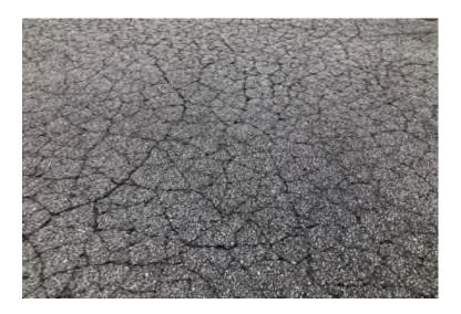
The typical method for making asphalt repairs is to saw cut and remove the damaged sections, check for and correct the underlying issue and then place new asphalt. It was noted that there are few repaired asphalt areas indicating that the pavement has performed well.
