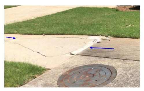
Replacement of damaged portions of curbing is covered by this category. Curbing repairs can be done with the rest of the **Masonry Rehab** repairs or can be done during repaving or asphalt repair projects. The portions of the curbing that are painted need to be repainted, and this is included in the **Asphalt Repairs/Seal-coating** category.
