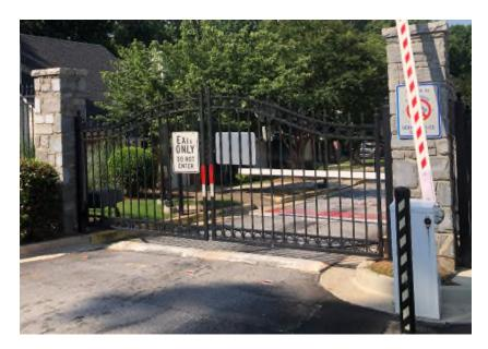
The swing gate operators have battery backup but as the operators age, the batteries lose efficiency and may fail. In addition, the new DoorKing operators no longer have built-in battery backup so a separate unit, called an Inverter, must be added at a cost of about \$2200. There are other manufacturers of swing gate operators that do have built-in battery backup.
