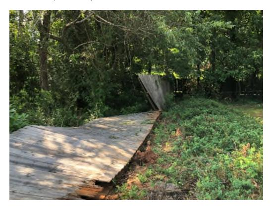
The 6-foot fence is less top-heavy and is generally still standing but has deteriorated and also damaged by falling tree limbs (see next photo).
