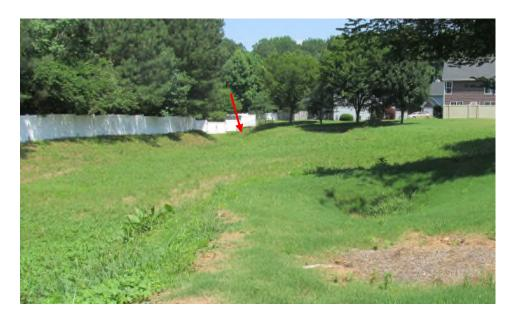
There is no inlet structure or outlet structure in that area but there is a normal drain at the low end of this area (the location is indicated by the red arrows in the previous and next photos) that collects the stormwater and then pipes it into the detention pond. The next photo shows a closer view of that drain just outside of one of the gates into the detention pond.
