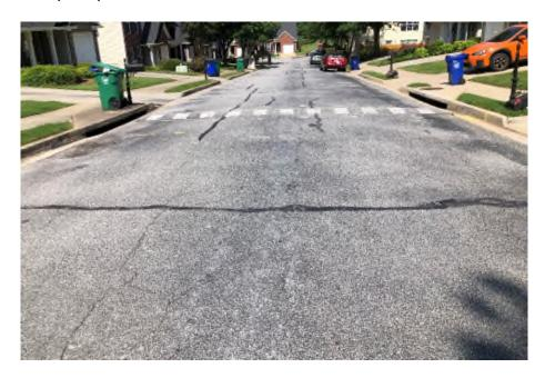
The typical construction of a street is compacted soil with four to six inches of well compacted base (i.e., crushed granite) and then asphalt layers totaling three to four inches. The durability of asphalt is determined at least as much by the strength and stability of the soil and base as it is by the quality of the asphalt pavement. The streets at The Gates at Bouldercrest are in good to
