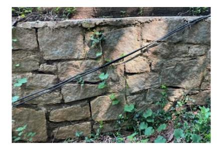
Part of the stone fence structure is leaning due to inadequate support. Funding is included in 2024 to correct this.
